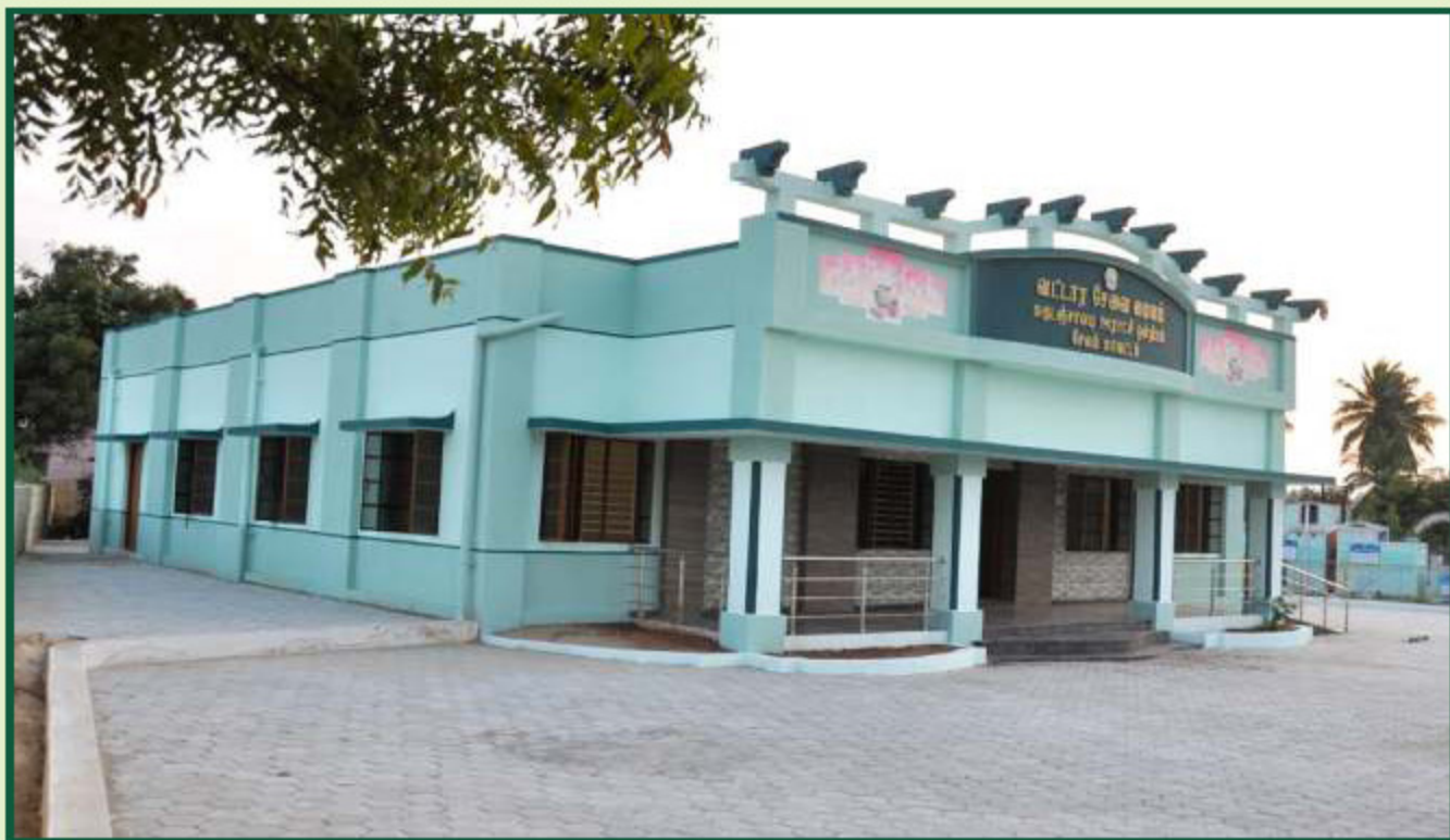
New Block Service Centre Building
