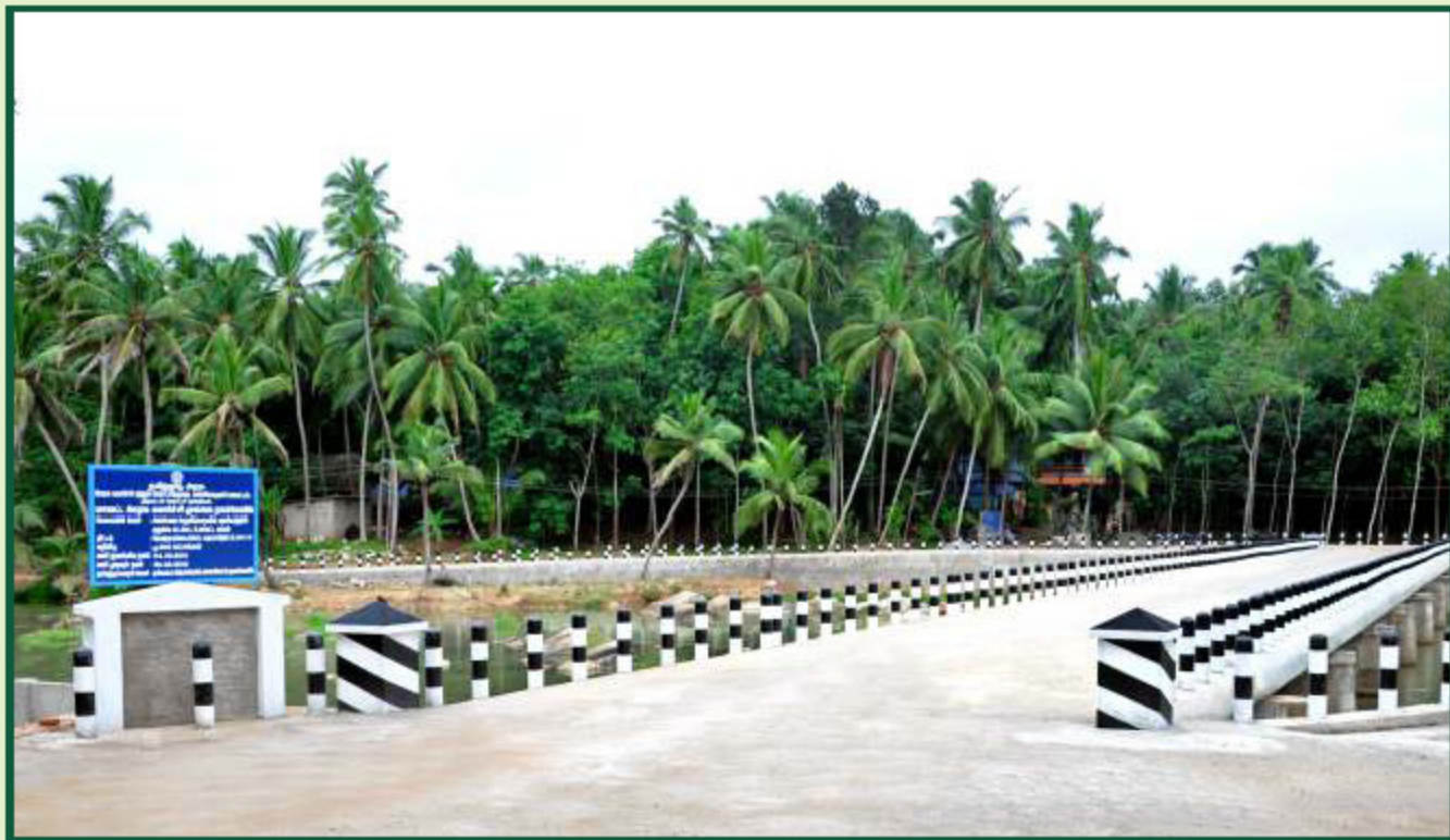
Construction of New Bridge
