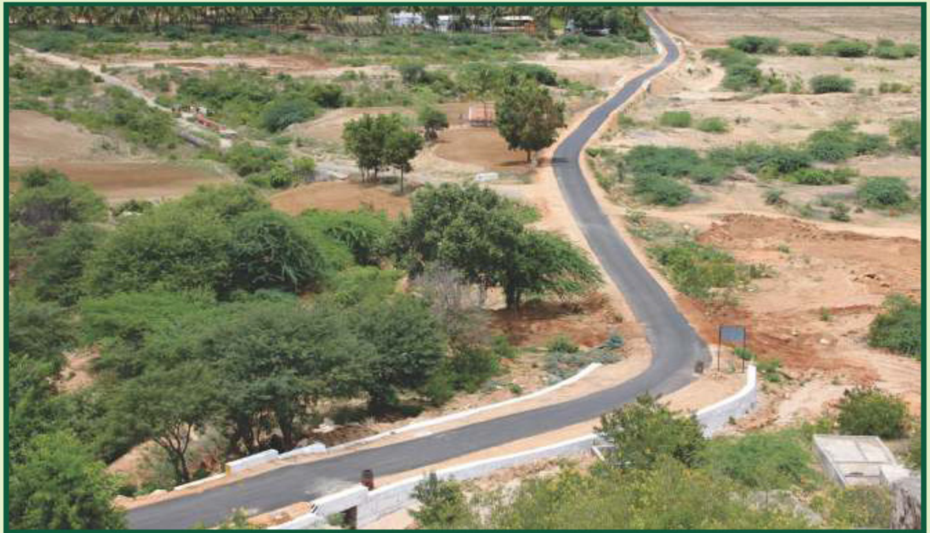
Formation of Black Topped Road
