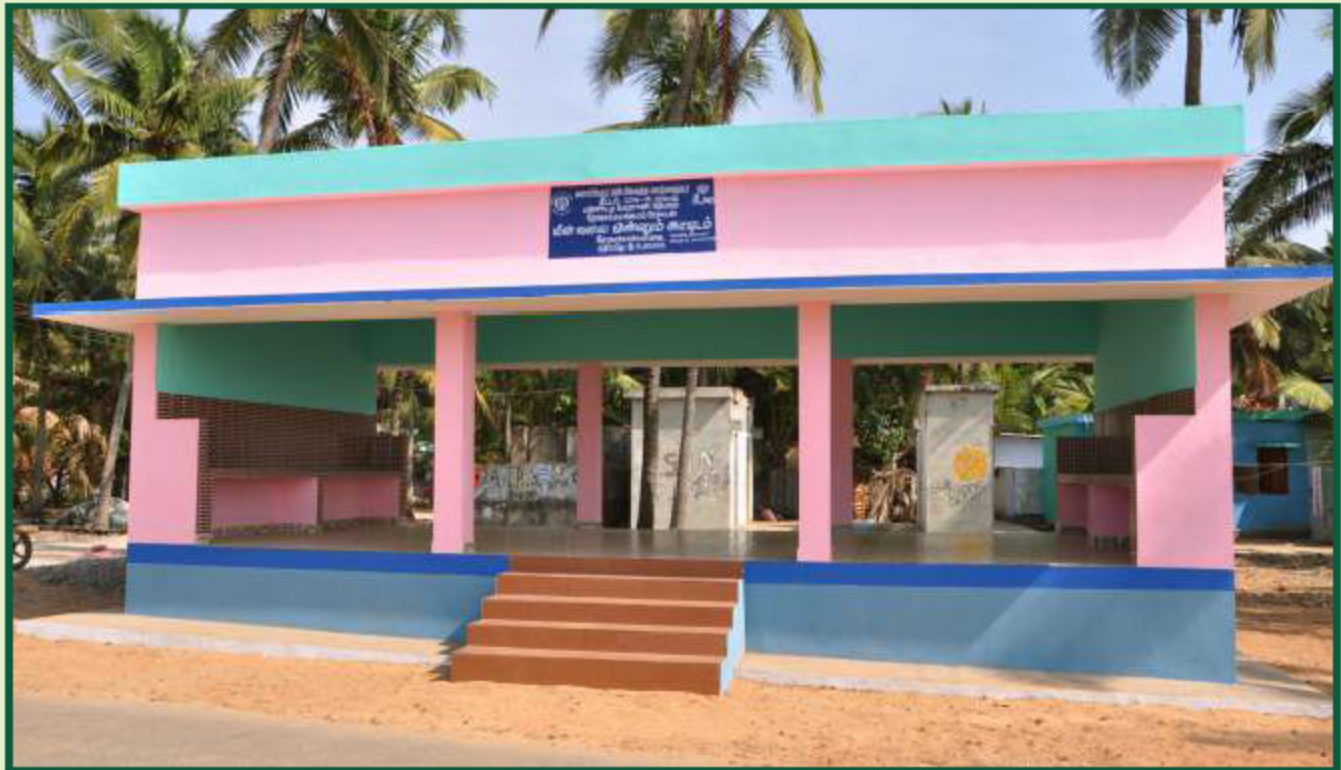
New Net Mending Shed under Post Tsunami Sustainable Livelihood Programme
